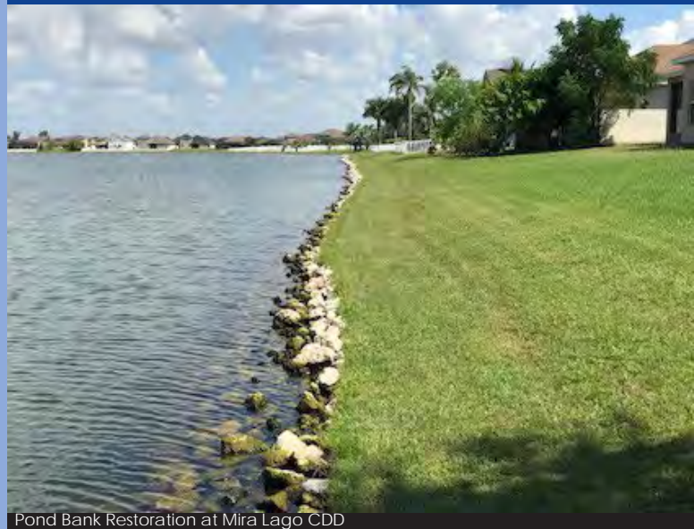
Pond Bank Restoration at Mira Lago CDD
