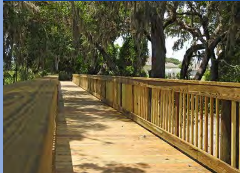
Pedestrian Boardwalk at Oak Creek CDD
