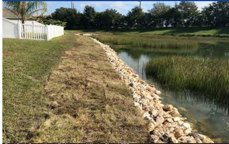
Pond Bank Restoration at Bridgewater of Wesley Chapel CDD
