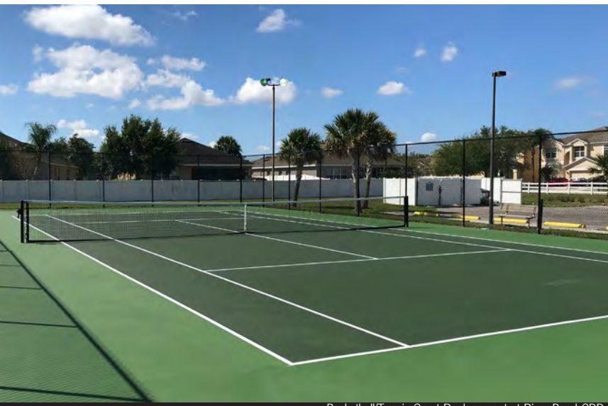
Basketball/Tennis Court Replacement at River Bend CDD
