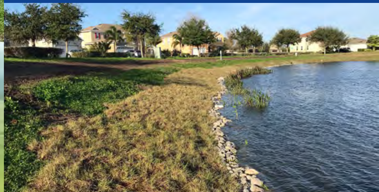
Pond Restoration at Harbour Isles CDD
