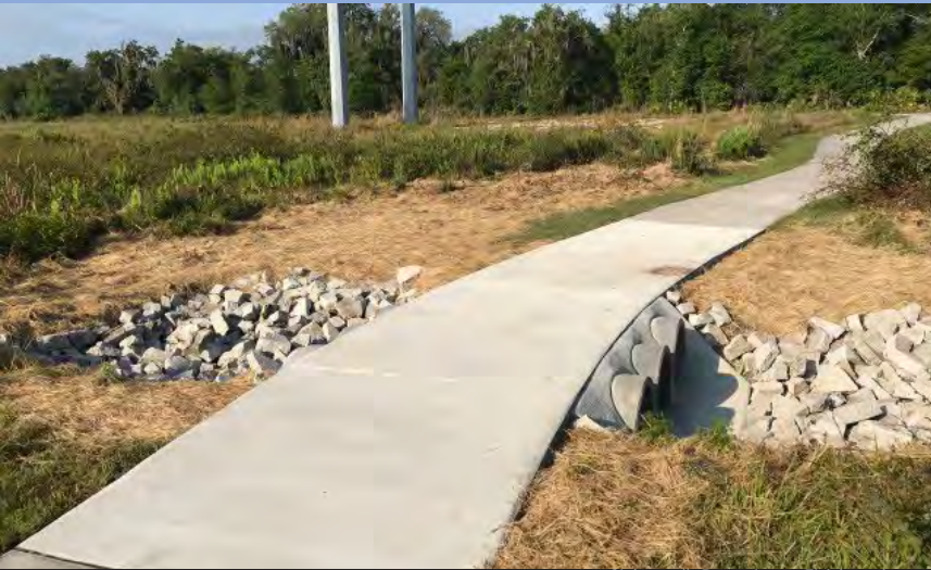
Sidewalk Repairs at Fishhawk Ranch CDD
